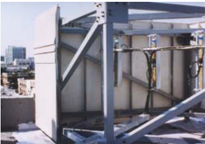
EXTREN® fiberglass plate and structural shapes were used for cellular shielding and were made to match the style and appearance of the Santa Ana Historical building.
