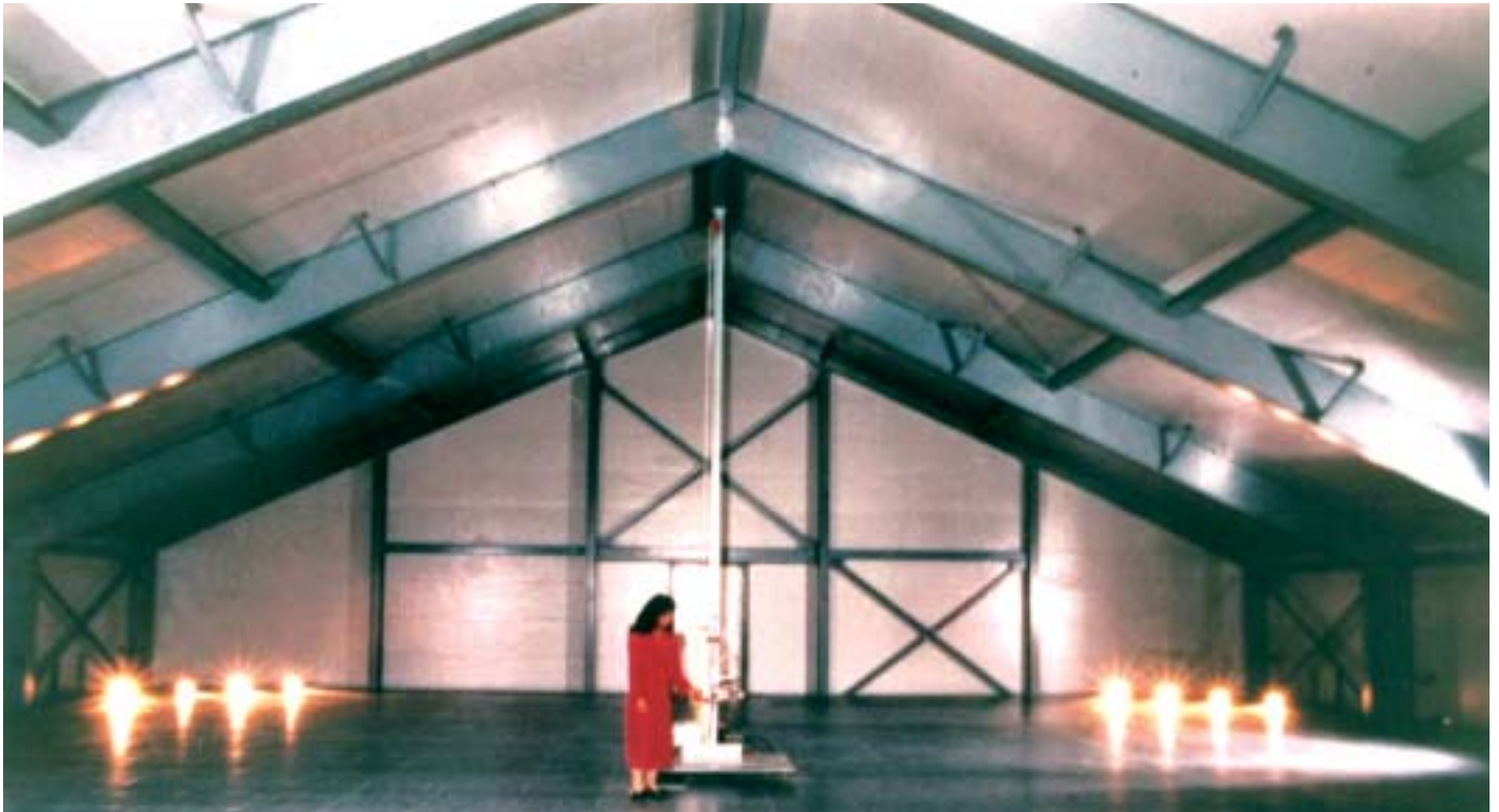
24" EXTREN® fiberglass I-beams span 62' wide rigid gables that support the siding and roof of an all-fiberglass building used for computer testing.
