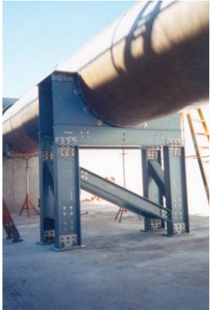
EXTREN® structural shapes were used to fabricate pipe supports to hold 1,000 lineal feet of 54" diameter pipe.
