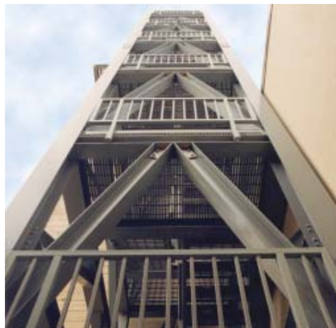
63' high freestanding fiberglass stair tower at Ft. Story Army Base, Virginia Beach, Virginia.
