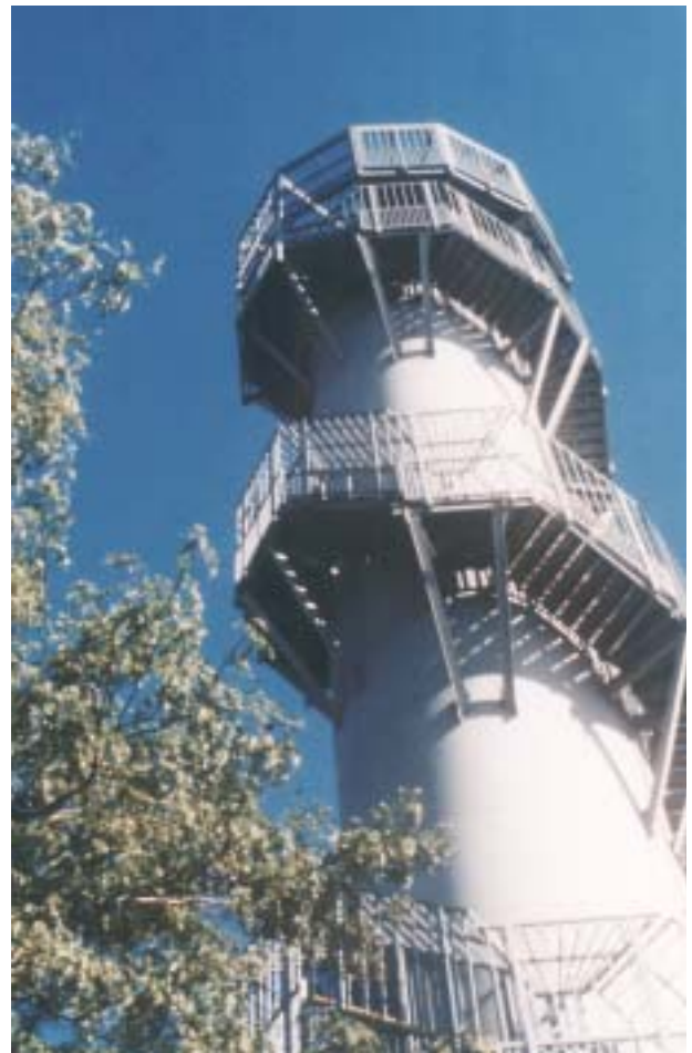
A system of FRP spiral stairs and landings circle the Cordova Park Observation Tower at Red Rock Lake near Des Moines, Iowa.
