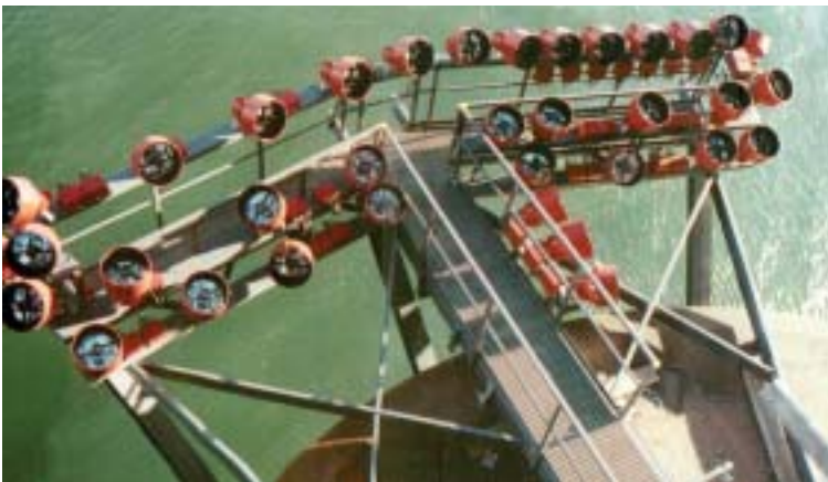
EXTREN® structural shapes were used to fabricate twelve platforms holding the spotlights that illuminate the Forth Bridge in Scotland.
