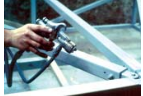
EXTREN® may be painted for better protection against long-term exposure to the sun.
