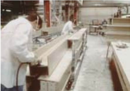
Beams are prepped before bonding connections together.
